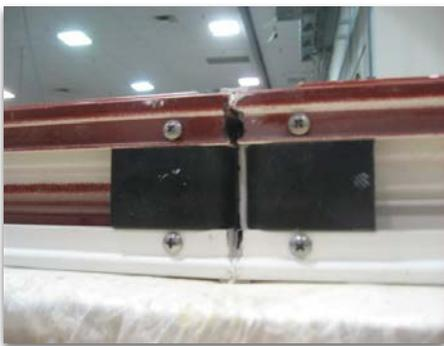
Clear adhesive can be used prior to inserting secure plate on both sides of the structural mullion to keep the plate in place until the window is set in the opening. Plate may be turned to interior or exterior depending on application.
