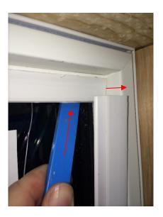
6.) After tucking the breather tube behind the glazing bead, use the rubber mallet starting from the bottom where the glazing bead groove that we disengaged from the top is still attached to the frame. Lightly tap the glazing bead at an angle with the mallet, following the bead to the top of the frame, until it snaps back into its original factory-set position.
