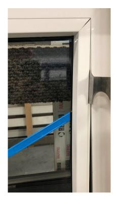
3.) Finally, use a rubber mallet to re-secure the glazing bead to the window frame. Gently tap the glazing bead at a 45° Angle until it snaps back into place. The easiest way to do this is to start tapping the mallet where the glazing bead is already installed into the frame and work your way UP/DOWN/LEFT/RIGHT.
