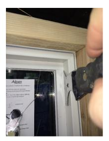
2.) Use gentle pressure, pressing the Five-in-One tool into the glazing bead between the frame and the glazing bead (being careful not to damage the finish). Apply the pressure as you wedge/slide the glazing bead out to the left away from the frame. This will allow the lip/groove that is on the glazing bead to separate from the frame, releasing pressure and allowing the glazing bead to detach/come loose.
