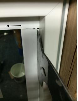
3.) Once you see the groove on the glazing bead has come out from behind the frame, set the Five-in-One tool or Plastic Folding Bone against the glass to get between the glass and glazing bead. Gently lever the glazing bead away from the glass, providing adequate room to tuck the breather tube behind the glazing bead (after it has been crimped properly).
