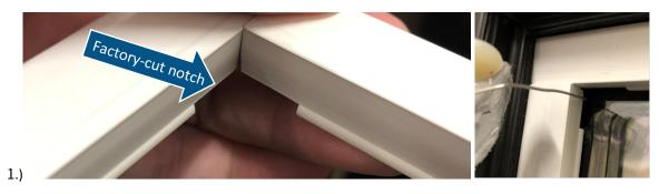
2.) Once the Capillary tube has been crimped and sealed properly, tuck/push the capillary tube through the channel that has been factory-cut into the glazing bead. Tucking the entirety of the capillary tube into this channel will allow the capillary tube to be concealed inside the glazing pocket.
