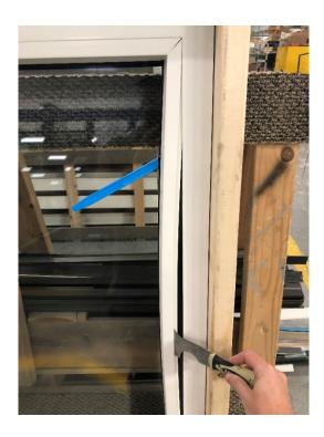
2.) Work your way UP/DOWN/LEFT/RIGHT with the 5-in-1 tool, gently levering the glazing bead away from the window frame (being careful not to damage the finish). Once the glazing bead has been released, use the plastic wedge to pry glazing bead away from glass, giving yourself enough room to tuck/hide/conceal the capillary tube.
